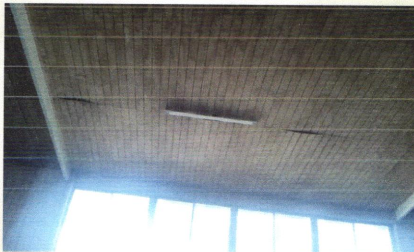
Interior techo comedor
