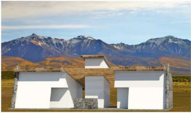
Vista Frontal Exterior
